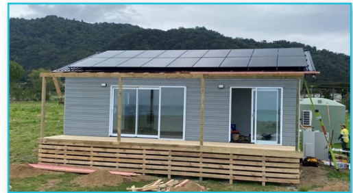
TMRE install team completing 5kw microgrid installation in Tauranga
