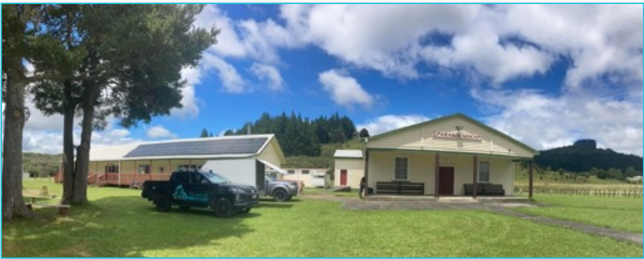
10kw Installation at Kaikou Marae, Pipiwai, Whangarei
