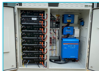
28.4kw of battery (+2x a Tesla Battery) on a 10kw inverter in Opotiki
