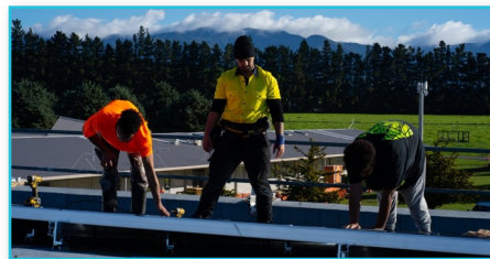
TMRE installing panels at Scanpower Dannevirke
