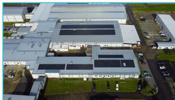
360kw installation at Scanpower, Dannevirke
