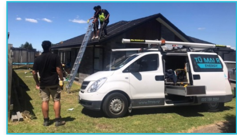
TMRE install team completing 5kw microgrid installation in Tauranga
