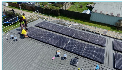
27.4kw Installation on 7 apartments in Gisborne
