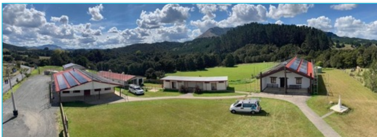
150kw installation at Tau Henare Marae, Pipiwai, Whangarei (largest solar array on a Marae in NZ)
