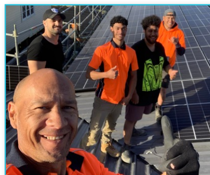
TMRE Team completing a 30kw installation at Whakapaumahara Marae in Whananaki
