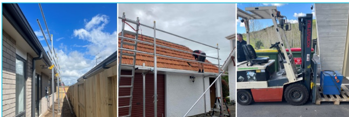
Far left: Scaffolding at Manawa. Middle: Platform at Whanganui. Right: Forklift at TMRE Office
