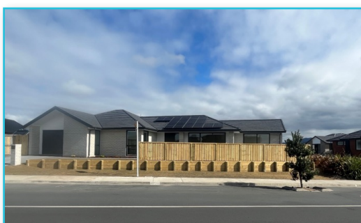
1 of 30 installations to be completed in Papamoa for Ngā Pōtiki
